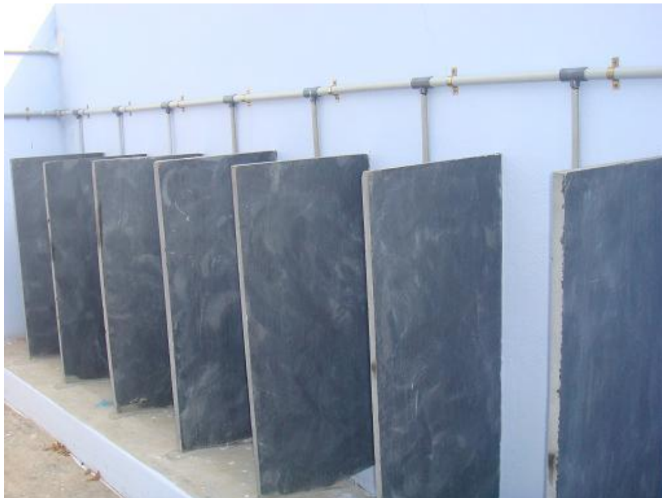
Toilet Inside View-1
